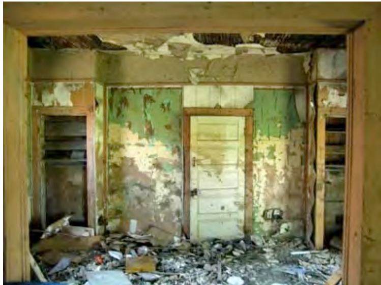
Inside of the original house before casting.
